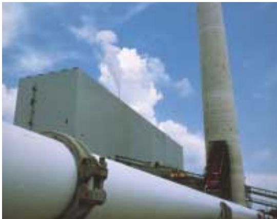
Plain end couplings provide full wall thickness joining for abrasive systems.
