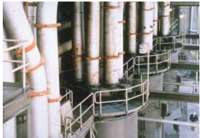
Severe services such as pulverized coal, fly ash slurry and others can be handled with stainless pipe and standard couplings.
