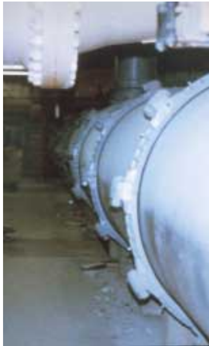
Large infalls/outfalls water treatment lines are easily assembled.
