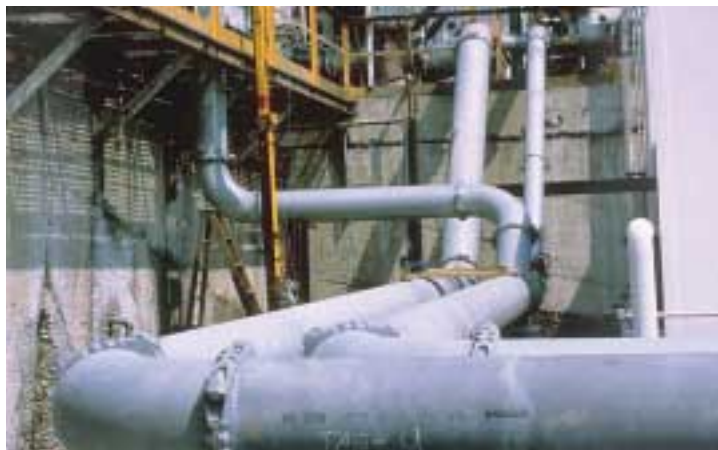
The grooved system provides products for black or galvanized steel, stainless, copper, aluminum, PVC, HDPE, lined/coated and specialty piping.
