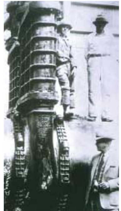
Large diameter valve settings have been common since the early 1930's.
