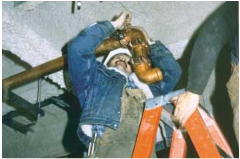
The copper connection for fast, easy, reliable pipe assembly without lead or flame.
