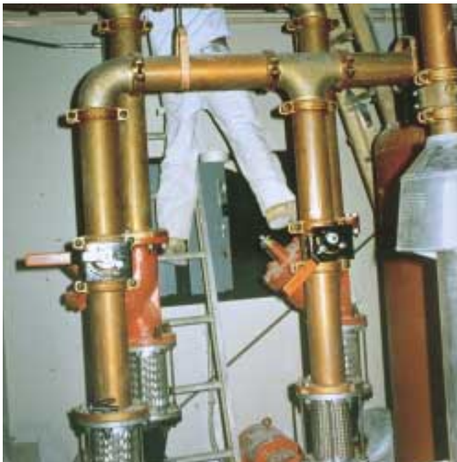
A complete package of copper (CTS) couplings, fittings, flange adapters and butterfly valves.
