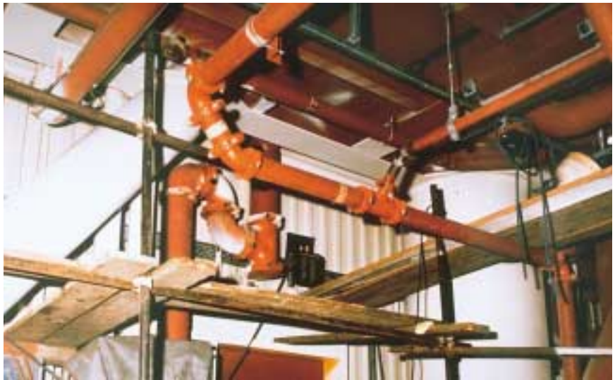
Special processes and unique configurations are easily assembled with the grooved system.
