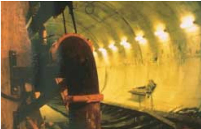
The grooved system eases tunnel piping, absorbs vibration and accommodates thermal movement.
