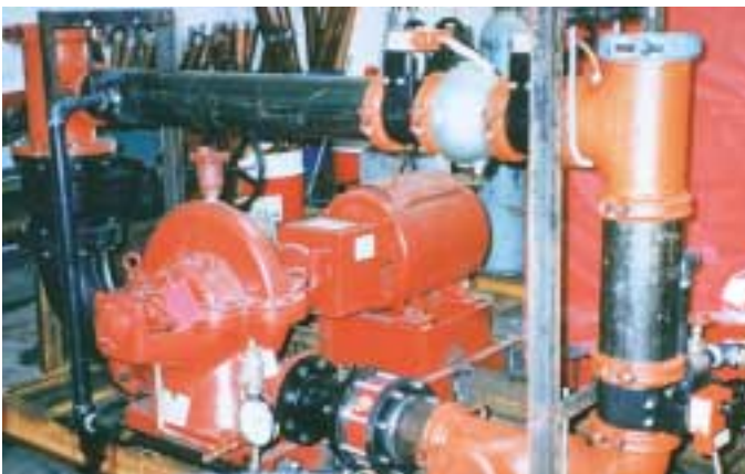
Pre-assembled fire pumps and other fire equipment utilize the complete system.
